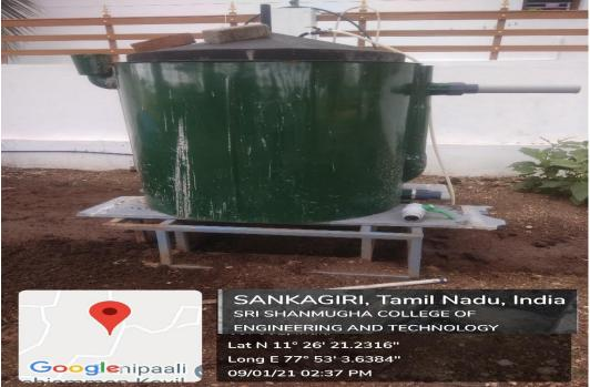
**Biogas plant:** Food Waste and Cow dung waste is converted into biogas and used as cooking fuel in the hostel mess. The capacity of the biogas scrubber plant is **900 liters.**
